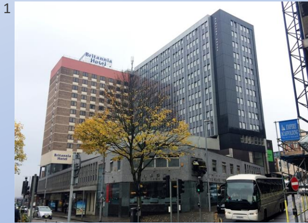
1 Newtown House, 1015 units, 2015-2016 Renovation Mabec Properties
